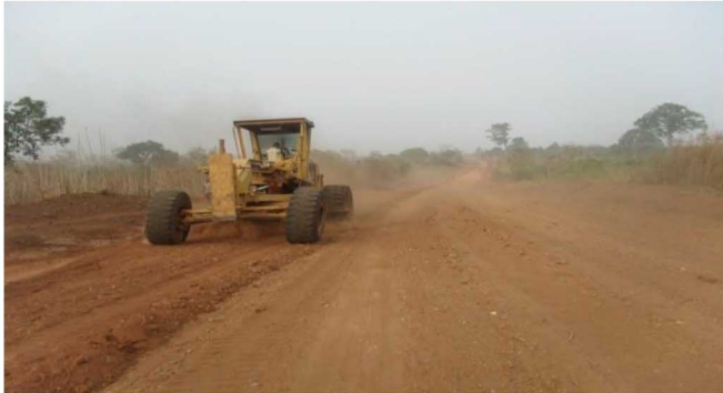
REHABILITATION OF KPANDO ROADS (25.64 ) VR 3
