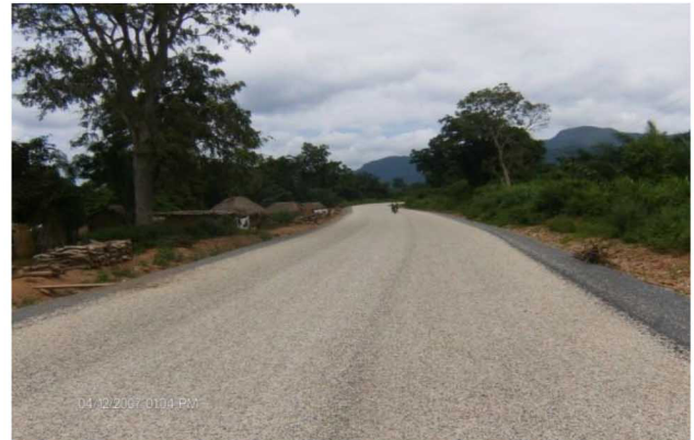
REHABILITATION OF KPANDO ROADS (25.64 ) VR 3
